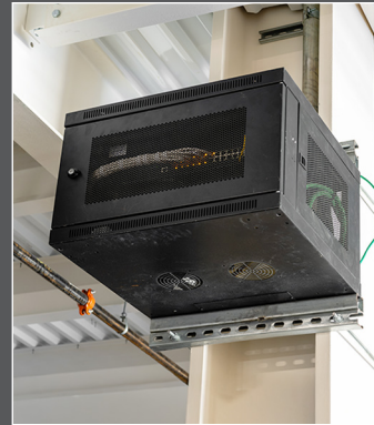
Each of Sinclair Digital's AGILE-CORE BITS distribution enclosures provides PoE lighting with Remeë's PowerPipe™ Class 4 FMP hybrid cable connected to each LED fixture with up to 1,000-foot runs, covering 10,000 square-feet of warehouse space.
