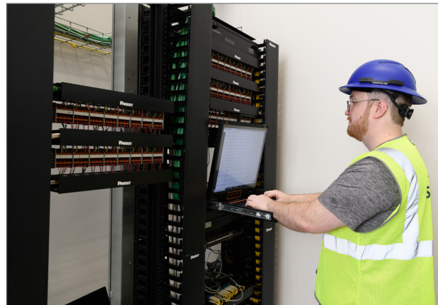
Reme's PowerPipe™ hybrid cable contains green jacketed copper cables the connect to the VoltServer transmitters, and a splitter feeds the yellow fiber cables to the switches.
