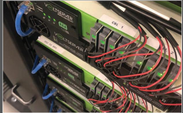
DE offers the convenience and safety of low-voltage distribution architectures such as Power over Ethernet (PoE), with the power and distance capabilities of traditional AC distribution.
