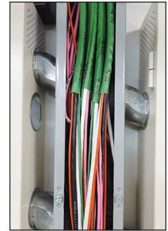
Cable pulls were reduced by 80%, as demonstrated in this cable tray containing the three main warehouse door composite cables.
