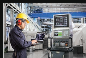
Industrial Control Station
