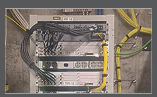
VoltServer's DAS equipment in tunnel using Remee's rugged PowerPipe™ cable.
