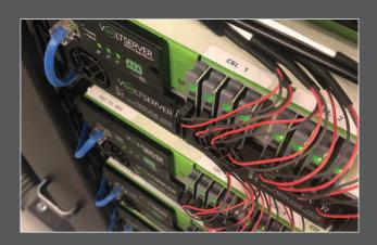
DE offers the convenience and safety of low-voltage distribution architectures such as Power over Ethernet (PoE), with the power and distance capabilities of traditional AC distribution.
